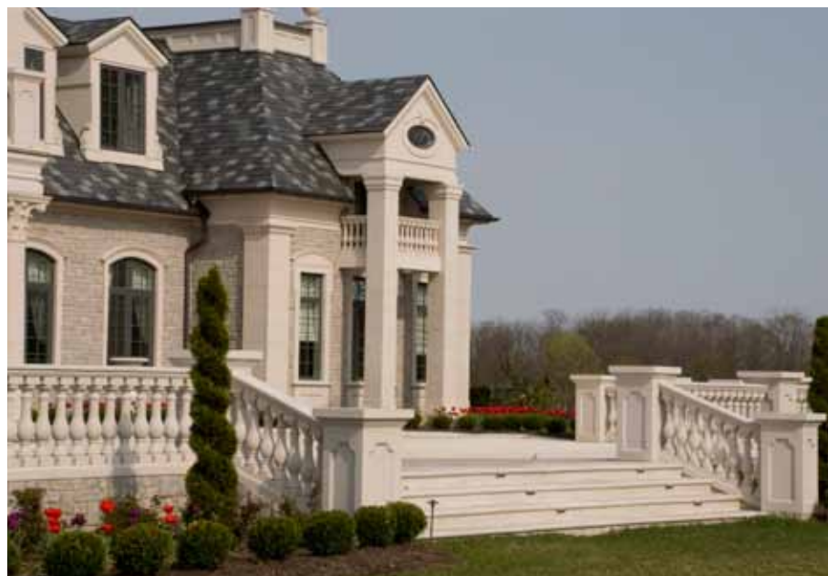
Custom and standard designs combine at this Ohio residence.
