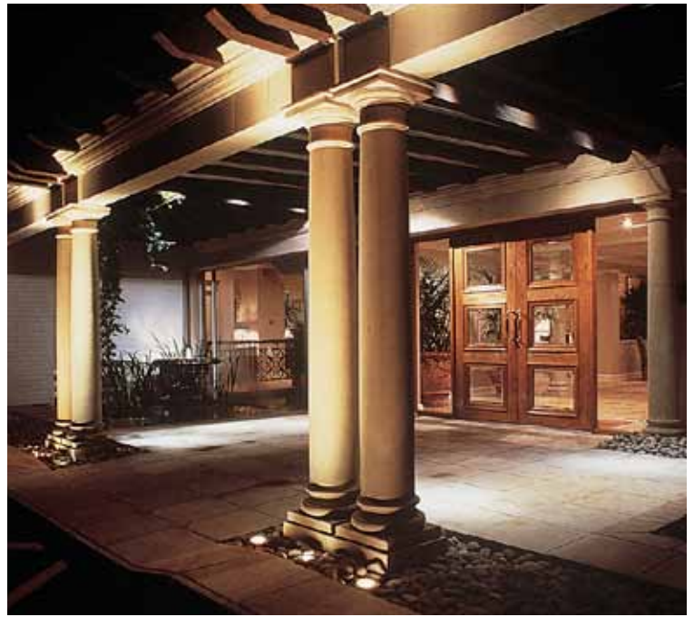
The entrance to the Atlantic Hotel, Jersey features Haddonstone columns.
