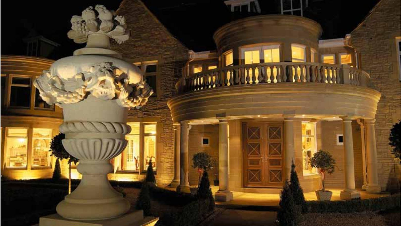
A private residence in West Yorkshire featuring a curved Haddonstone portico with balustraded balcony and a Mount Edgcumbe Finial in the foreground.
