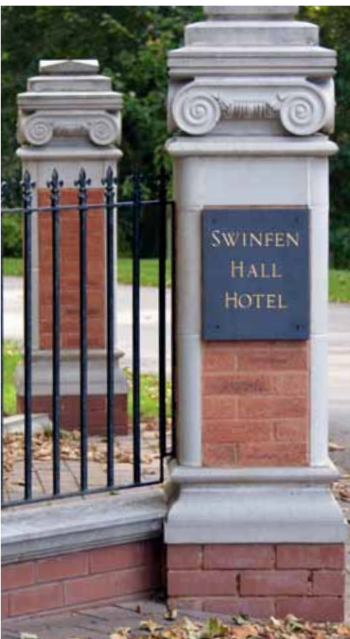
Bespoke gate piers at Swinfen Hall Hotel in Staffordshire.
